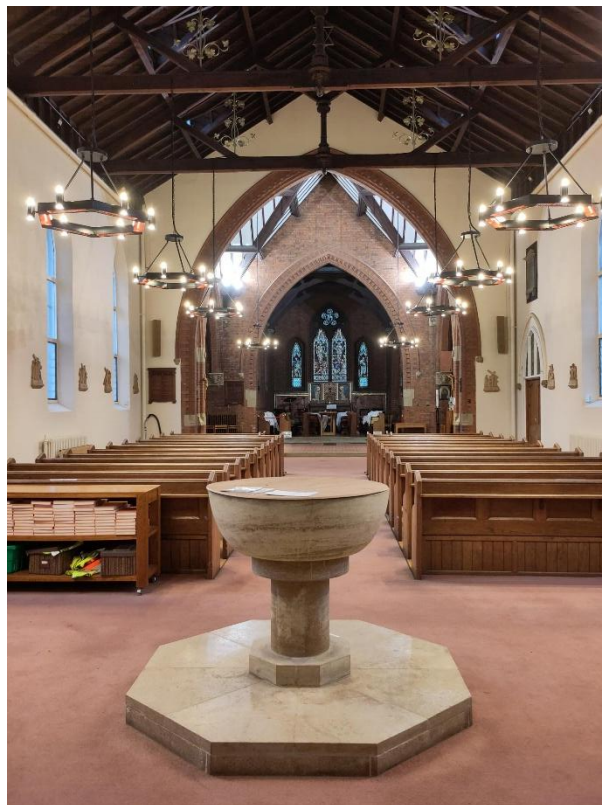
Day 3 Chandeliers installed in Nave
