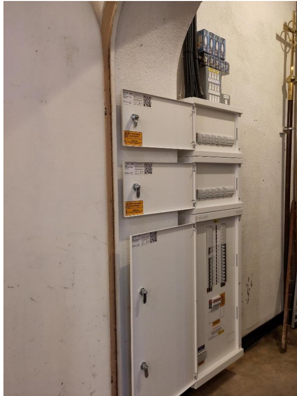
Day 3 Control cabinet complete
