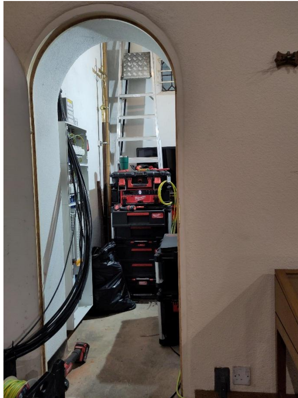
Day 2 Control box under construction
